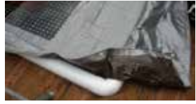
Detail of wash pit construction.
