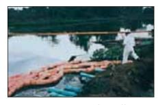
3M<sup>™</sup> Petroleum Sorbents are used extensively for controlling, cleaning up, and recovering oil and
