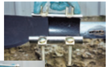
Just wrap bandage around pipe and tighten the clamp.
