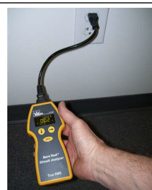
USE AC128 SURETEST CIRCUIT ANALYZER TO CHECK CIRCUIT LOAD
